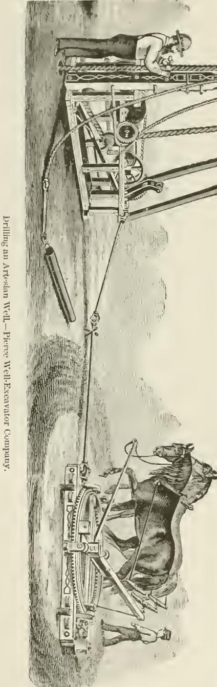
Drilling an Artesian Well—Pierce Well-Excavator Company.
